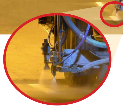
▲ A close-up photo of the truck spraying the lane markings
