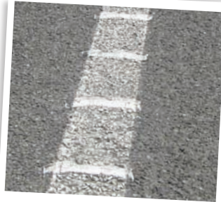
A rumble strip
