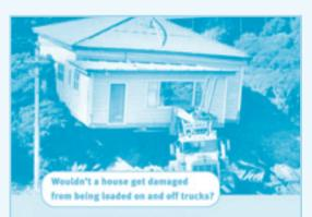
Houses built from wood are very flexible and can bend quite a lot. If a house is too wide for the road, it can be cut in half or thirds and moved in pieces. Then it is joined together again when all the pieces get to the new section
